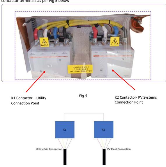
Recommended Cable Size: Main Cable - 70mm<sup>2</sup> x 4C, Earth Conductor - 50mm<sup>2</sup> x 1C
